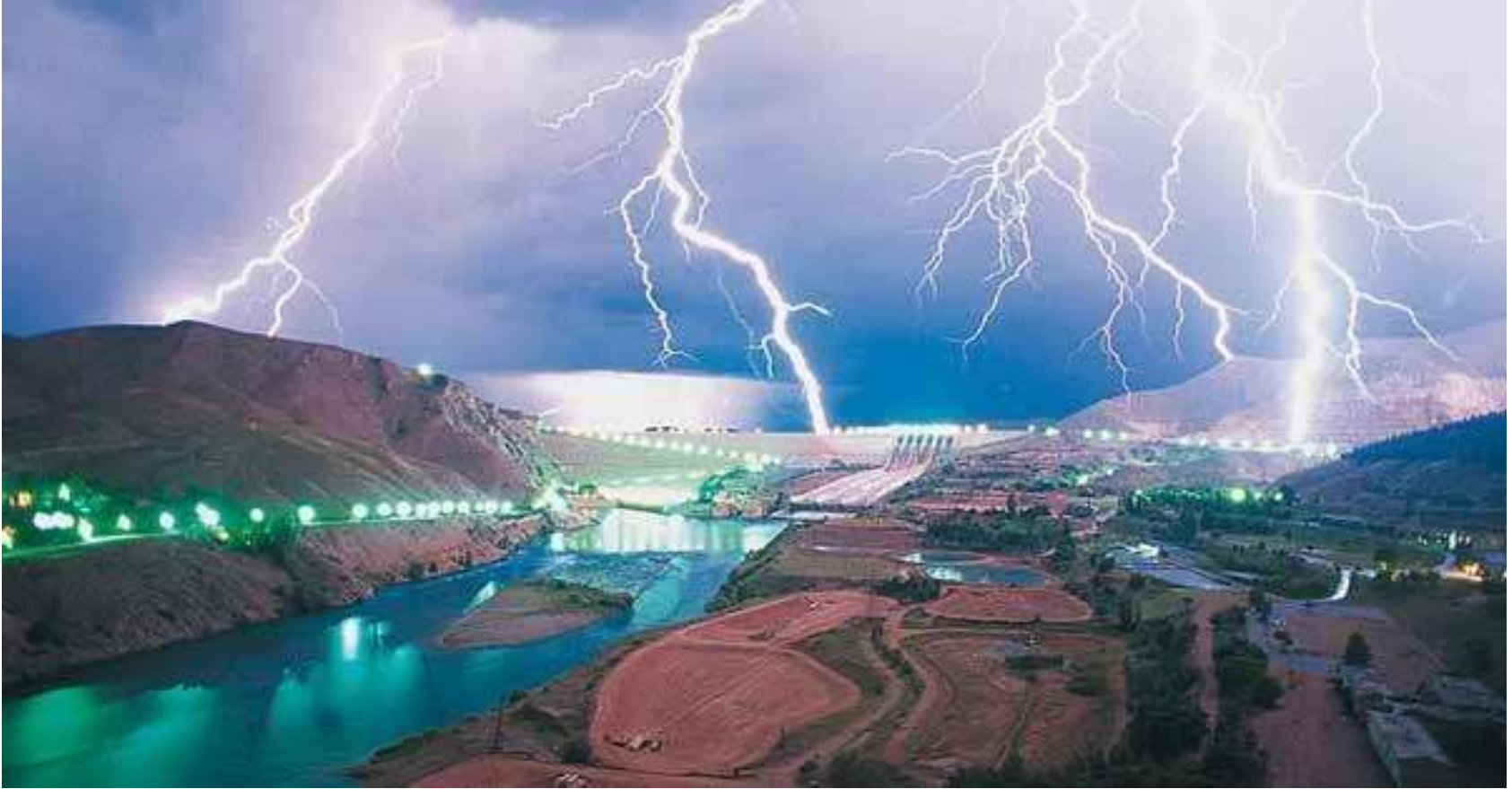
Keban Barajı/ Elazığ
