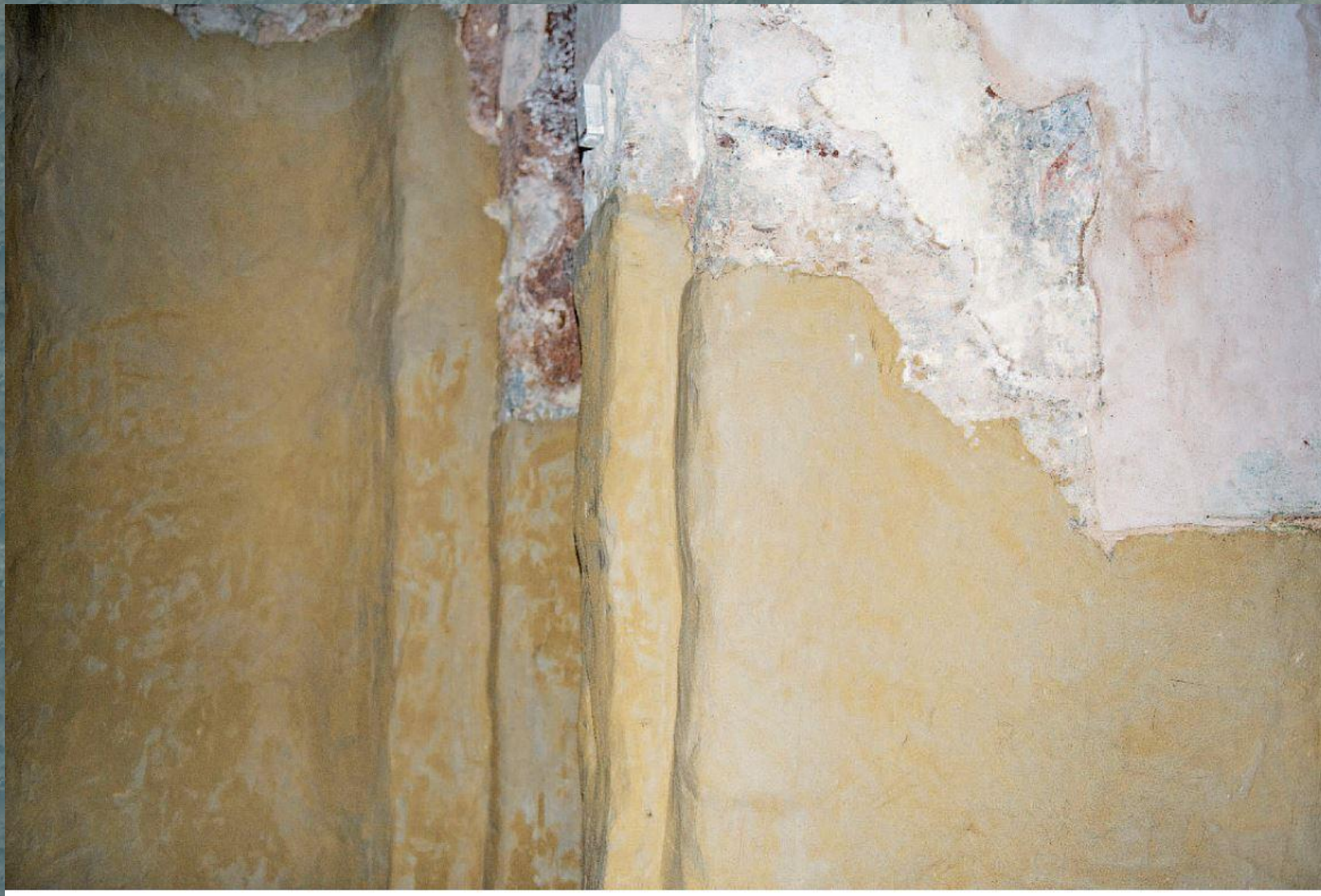
Sacrificial render applied to a wall within the church of St. Michael, Ston (Croatia), 11th century; Photo: 2011, HRZ (Veronika Šulić); Weyer, E. (ed.), (2015), EwaGlos: European Illustrated Glossary Of Conservation Terms For Wall Paintings And Architectural Surfaces , Petersberg: Hornemann Institute; 308.
