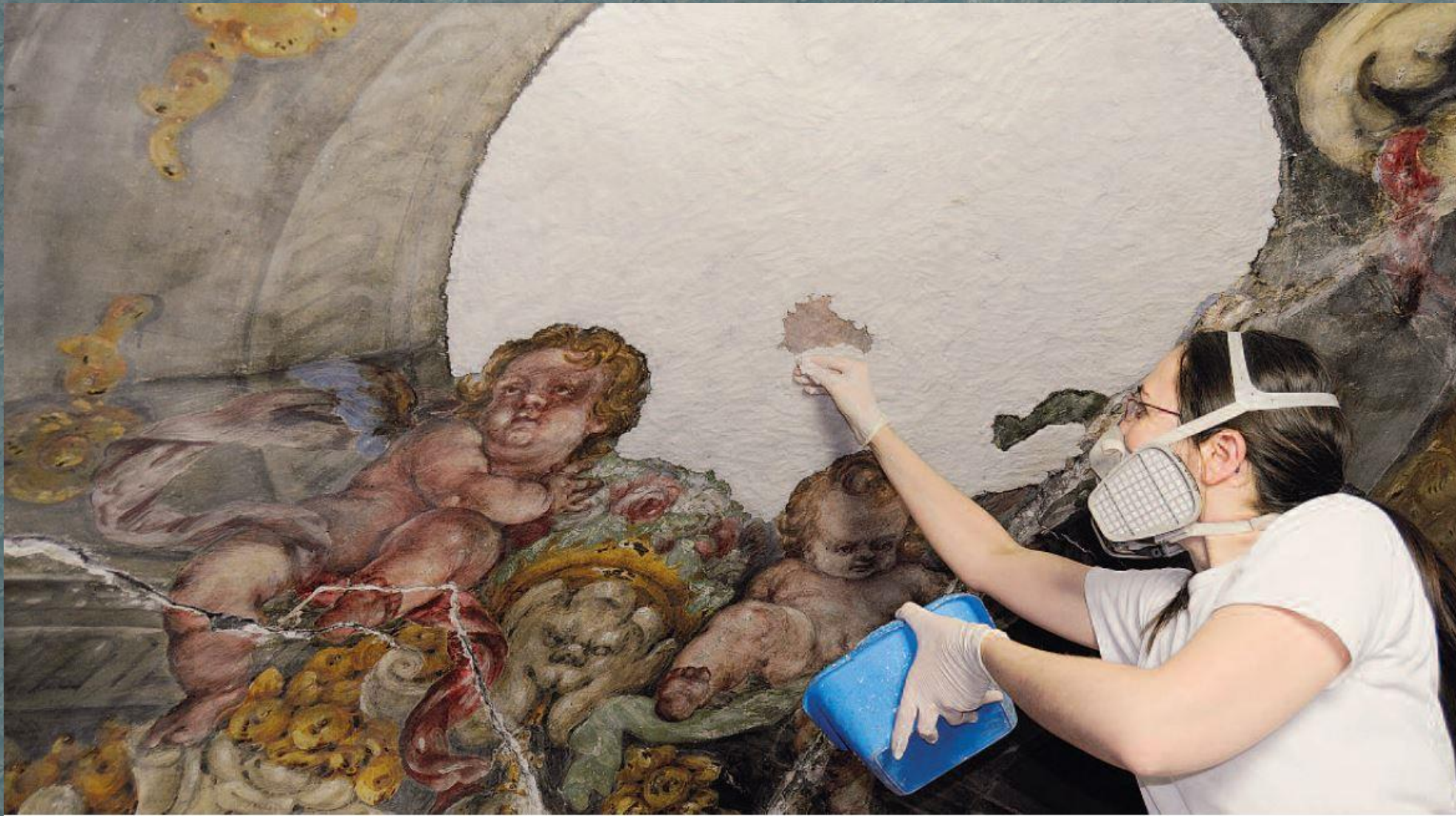
Application of a poultice, wall painting by Dionis Vidal, Church of San Nicolas Obispo y San Pedro Martir, Valencia (Spain), 1694-1700; Photo: 2014, UPV; Weyer, E. (ed.), (2015), EwaGlos:European Illustrated Glossary Of Conservation Terms For Wall Paintings And Architectural Surfaces, Petersberg: Hornemann Institute; 310.
