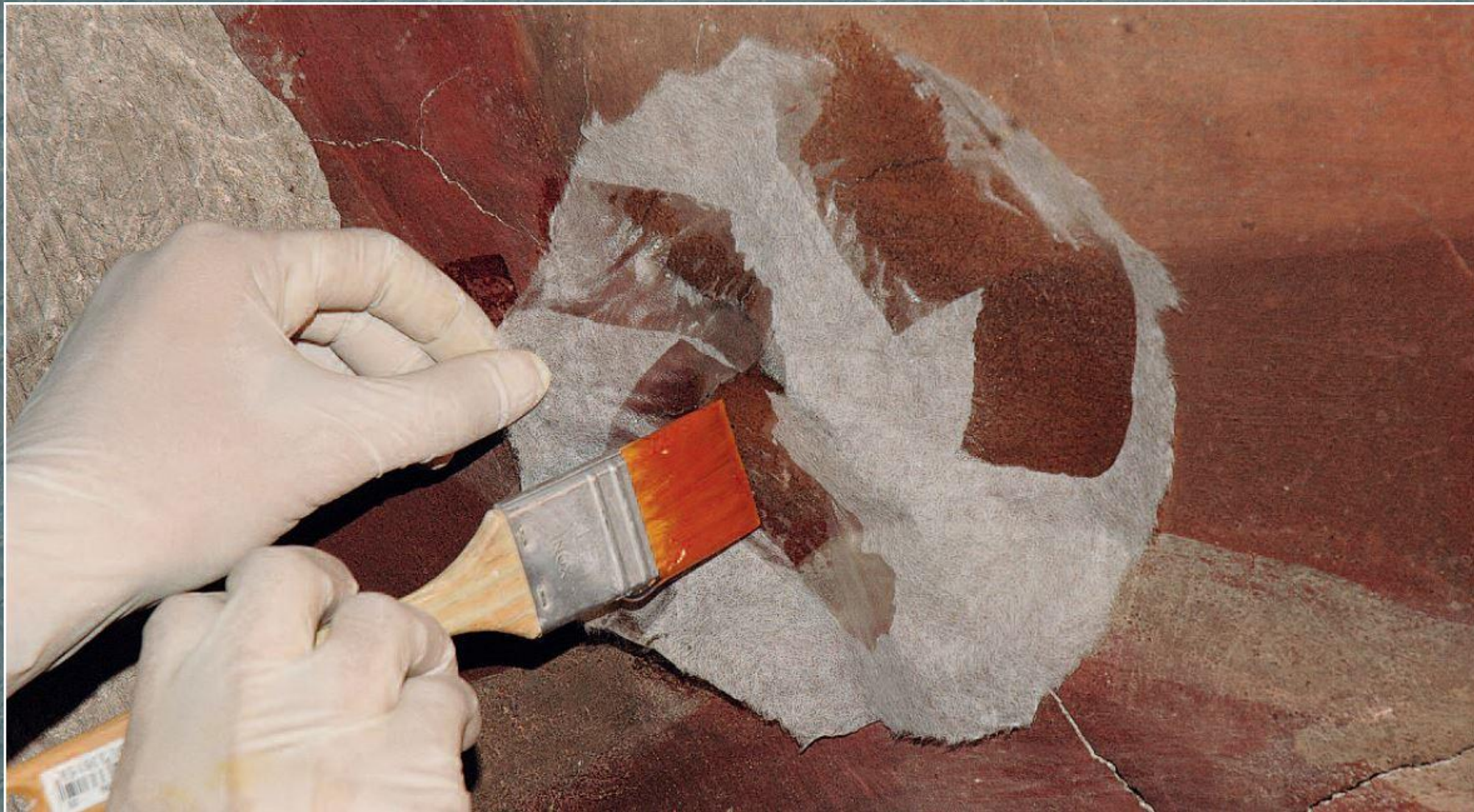
Application of a consolidant, wall painting by Antonio A. Palomino/ Guilló, Church of Santos Juanes, Valencia (Spain), 1698-1700; Photo: 2009, UPV; Weyer, E. (ed.), (2015), EwaGlos:European Illustrated Glossary Of Conservation Terms For Wall Paintings And Architectural Surfaces , Petersberg: Hornemann Institute; 312.
