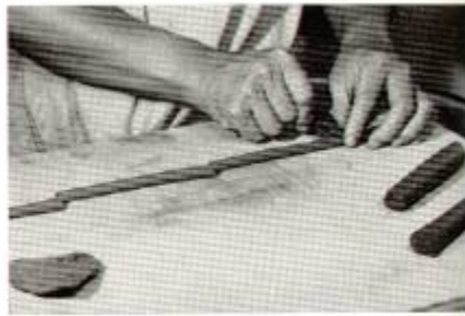
FIGURE 50. The clay is cut to equal lengths.
