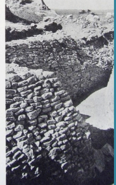
189 Tower R from East, Showing Bulge in Sides
