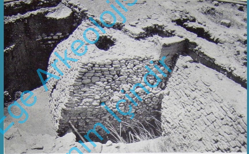
189 Tower R from East, Showing Bulge in Sides
