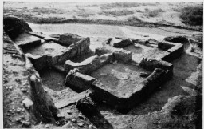
e. The 'Residence', with Room 180 (Fig. 79) in the foreground; cf. p. 138
