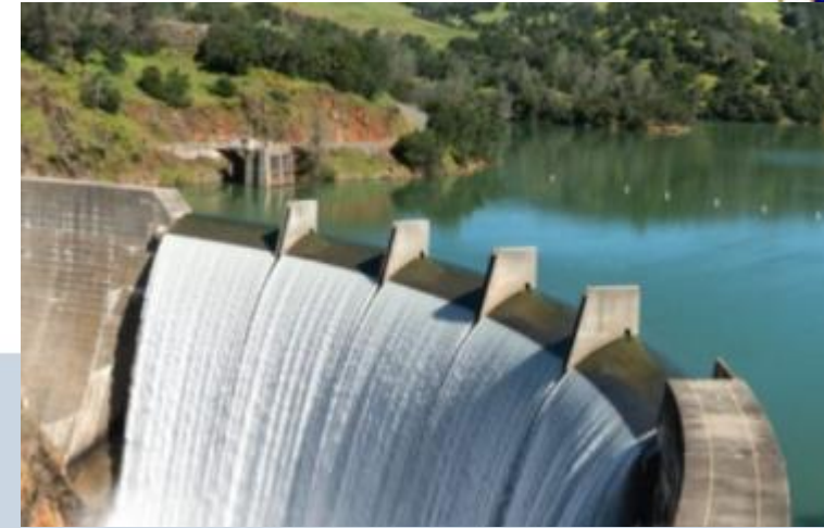
Hydroelectric power plant
