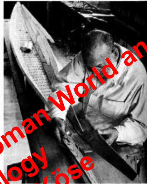
Reconstructing the oldest ship in the world. In 1954 the charred remains of parts of a centuries-old boat were found buried in a pit on the south side of the Great Pyramid of King Cheops at Giza, Egypt. (Top left) An important clue to the reconstruction proved to be the four classifying signs carved on most of the timbers that indicated in which of the four quarters of the ship the timbers belonged. (Right) Hassan Ali Youssef used a planimeter to help in the work of reconstruction. (Left) After 14 years of work, 1244 pieces of the hull were finally reassembled.
