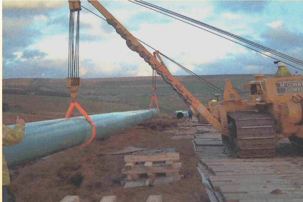
Working over trackmat without topsoil/turf stripping
