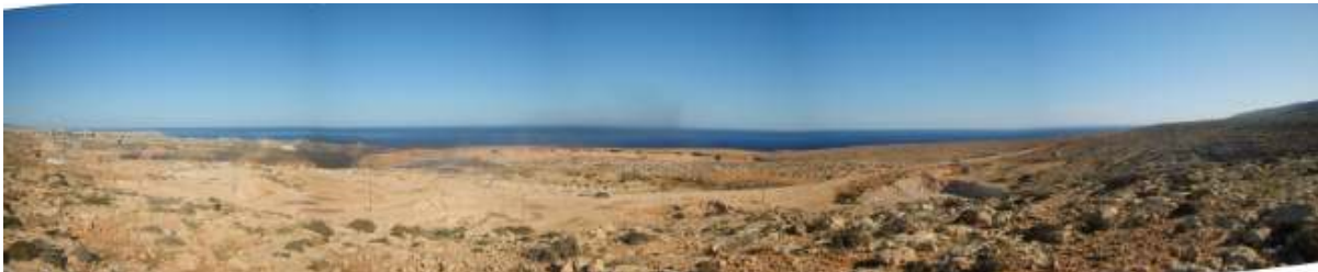
Fig. 9: The solid waste open dumping area at the east of the city, and the natural landscape that will be used for city development.
