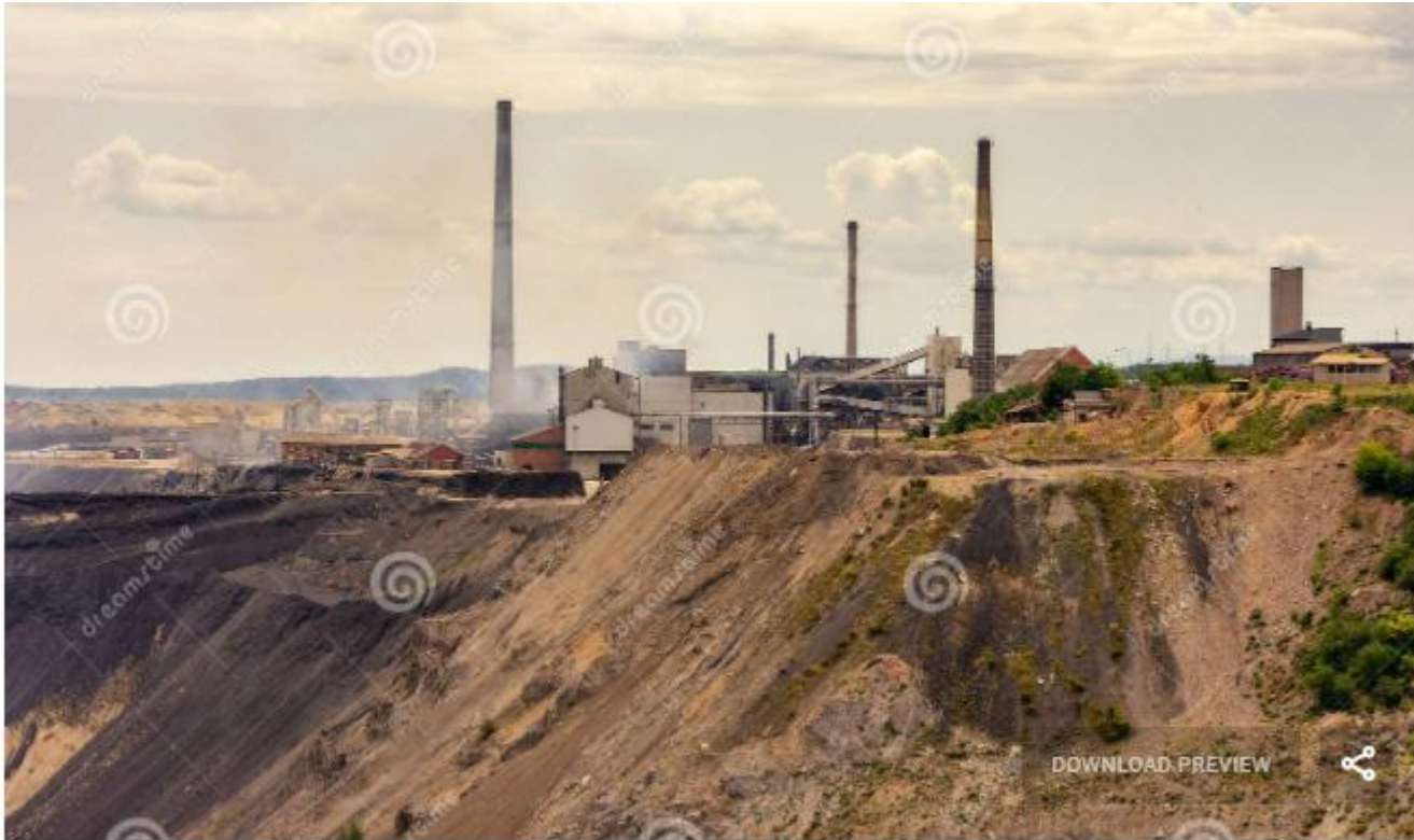
Bor / Serbia - July 13, 2019: Copper mine and smelting complex of Zijin Bor Copper in Bor, Eastern Serbia, one of the largest copper mines in Europe owned by Chinese mining company Zijin Mining Group
