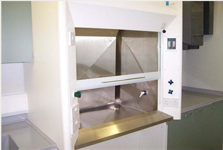
Fume cupboard suitable for use with radioactive materials
