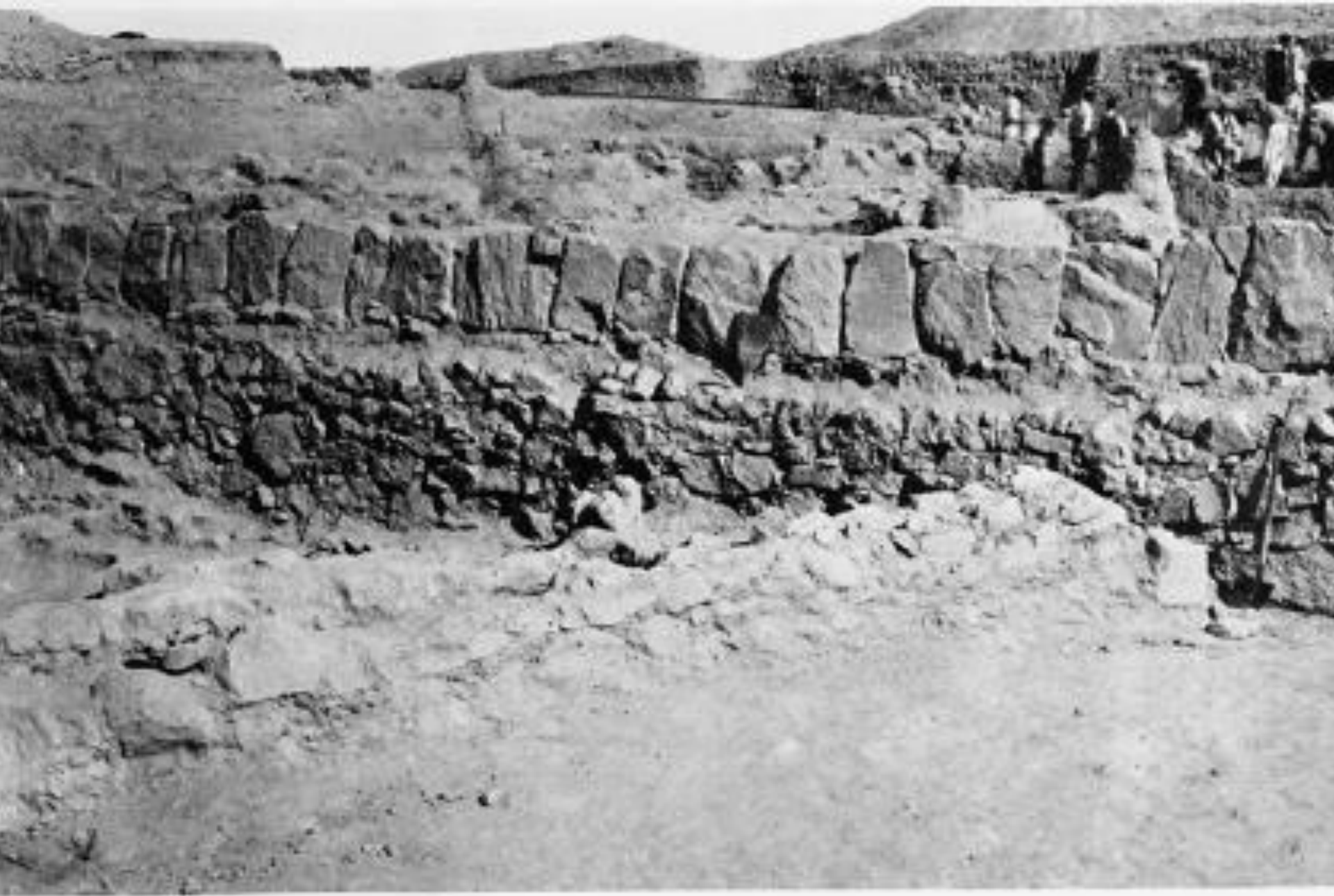
FIG. 10.—DADO SLABS ON THE SOUTHERN FAÇADE OF THE MANSION OF LEVEL 10 T
