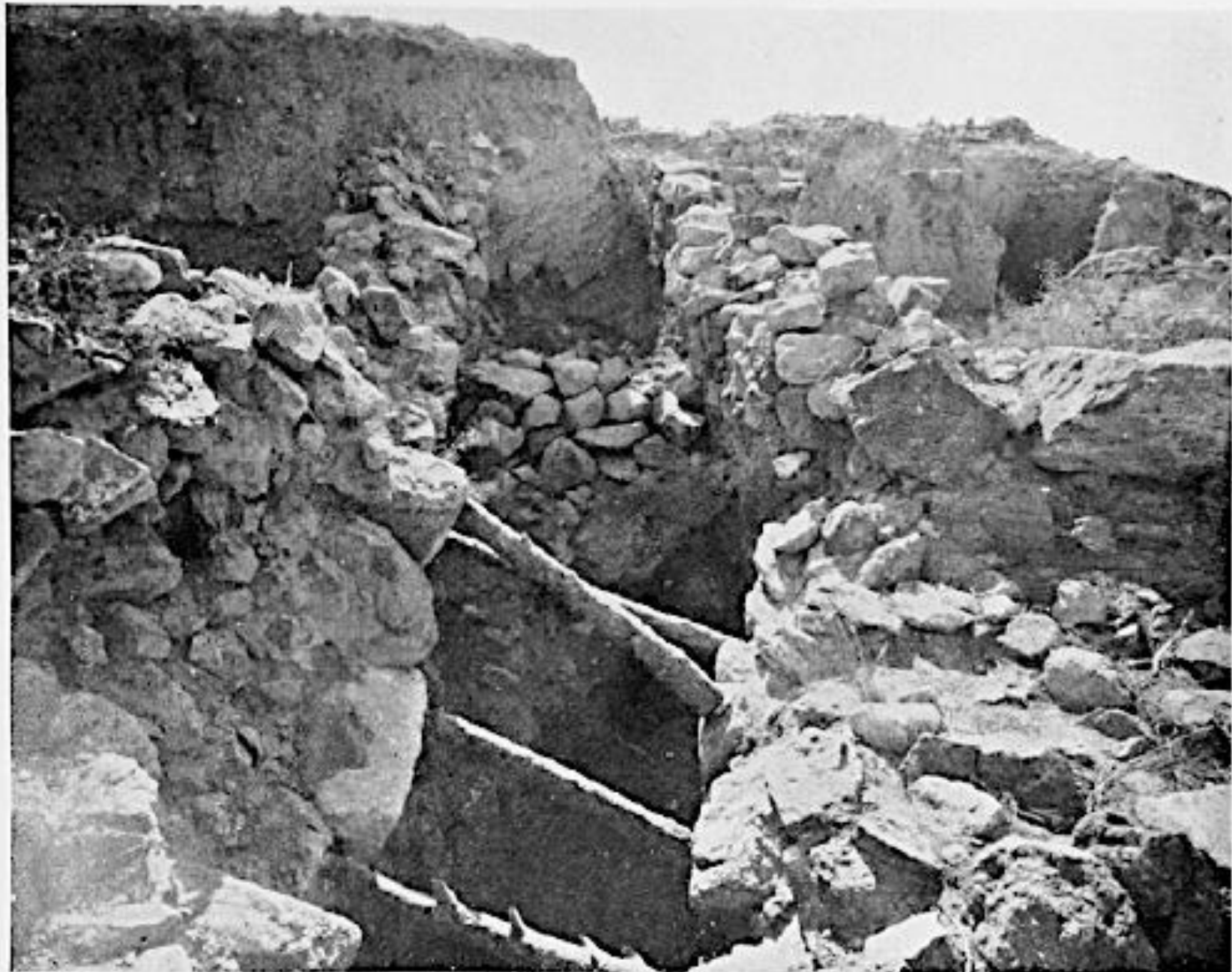
FIG. 31.—POSTERN FROM EAST-NORTHEAST, SHOWING NEW ENTRANCE CUT IN SOUTH WALL OF PASSAGE DURING PERIOD OF LEVEL 10 T
