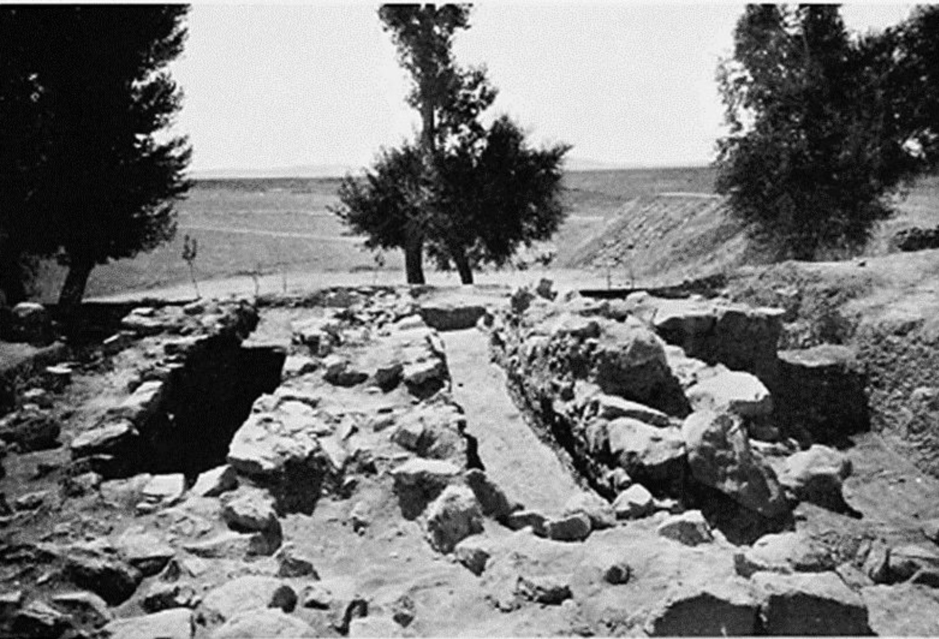
FIG. 91.—WESTERN TOWER OF SOUTHERN GATEWAY, FROM NORTH
