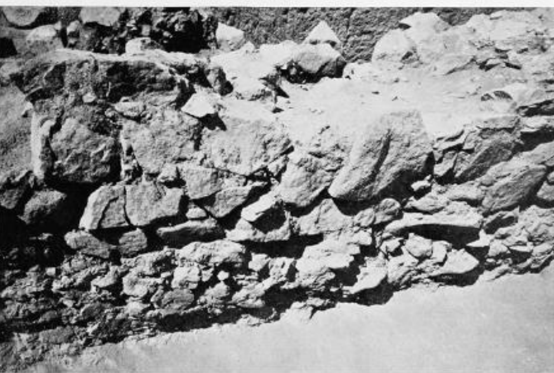
FIG. 5.—AN OUTER WALL OF THE WEST TOWER OF THE SOUTHERN GATEWAY IN LEVEL 10 T
