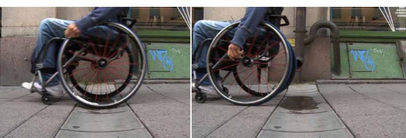
**"Flattening" the street** environment is another important means of improving access for wheelchair-users and parents with prams. Among other things, the City has replaced all pavement guttering – the channels leading water from downpipes across the pavements and into the street drains.
