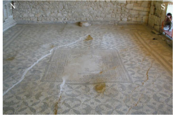
Figure 5. Normal faulting in the Neon Library (see Figure 3 for location).
