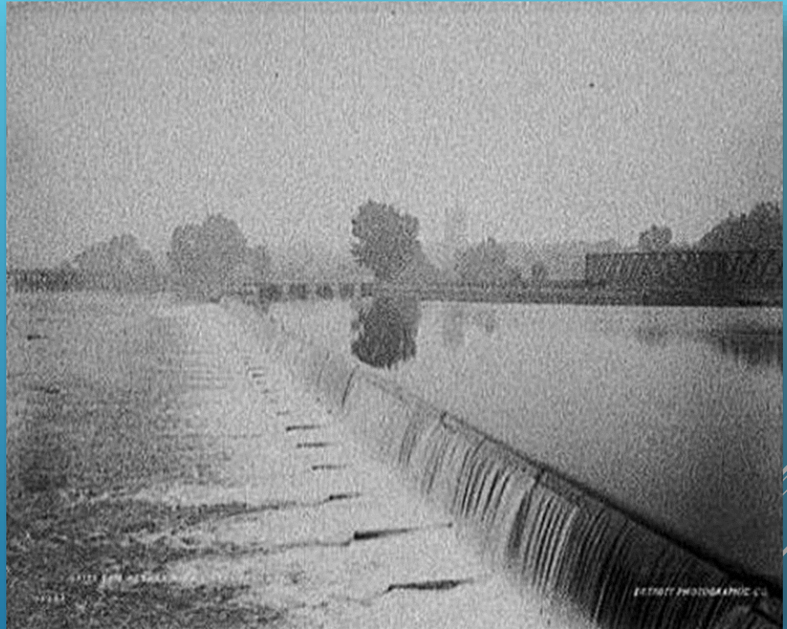
The dam across Fox River in Appleton, Wisconsin, the site of the first hydroelectric power plant in the world (1882).
