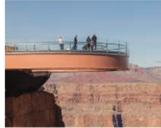
This cantilever support is fixed at one end and extends out into space at the other end.
