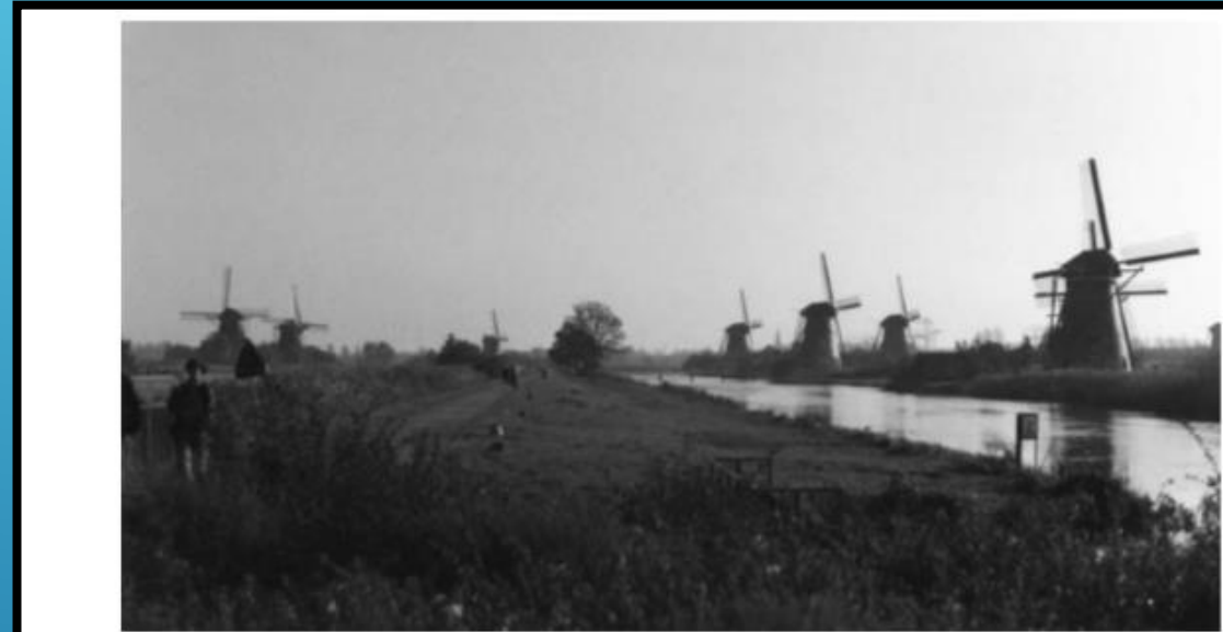
FIGURE 1.1 Dutch windmills, World Heritage Site, Kinderdijk, The Netherlands.
