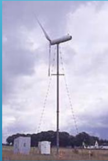
Guyed Pole Tower
