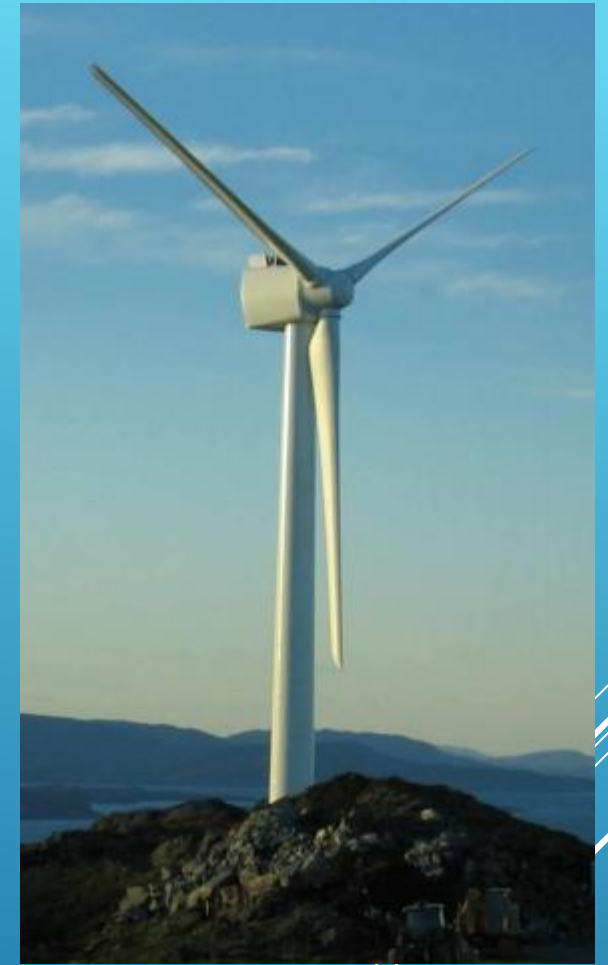
Tubular Steel Towers
