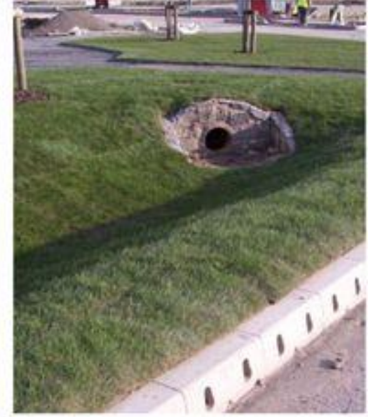
Maintaining a grass height of 50mm optimises primary filtration within the swale.
