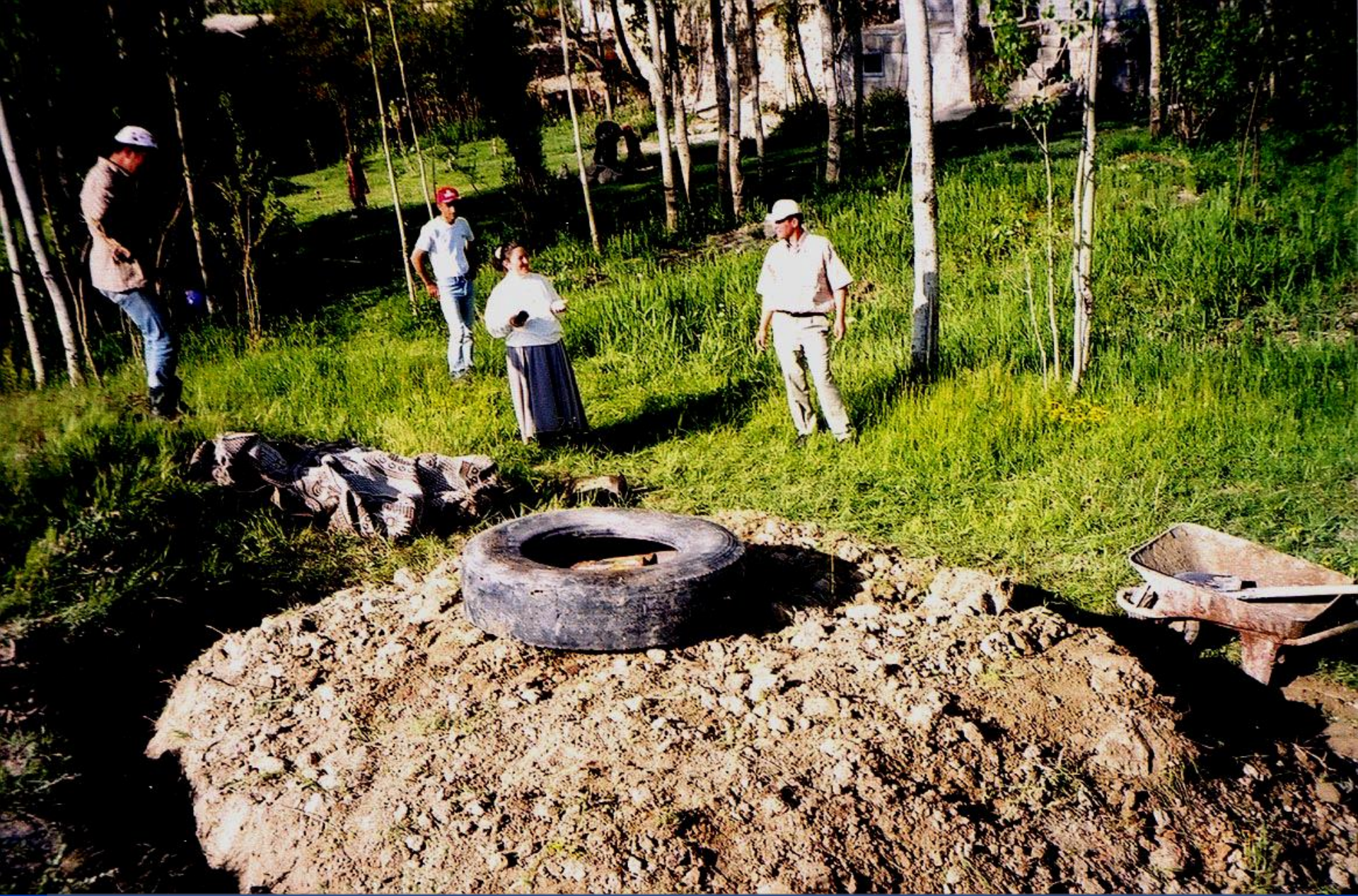
silo material left to stand by ditching around
