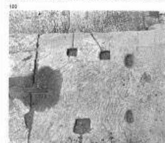
119 Wedging together blocks with a crowbar and clamping.
