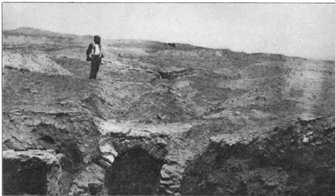
FIG. 15.—The Arched Sewer at Fara, Built of Plano-Convex Brick.
